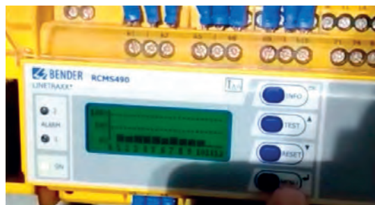
LINETRAXX® Residual current monitoring system RCMS490
