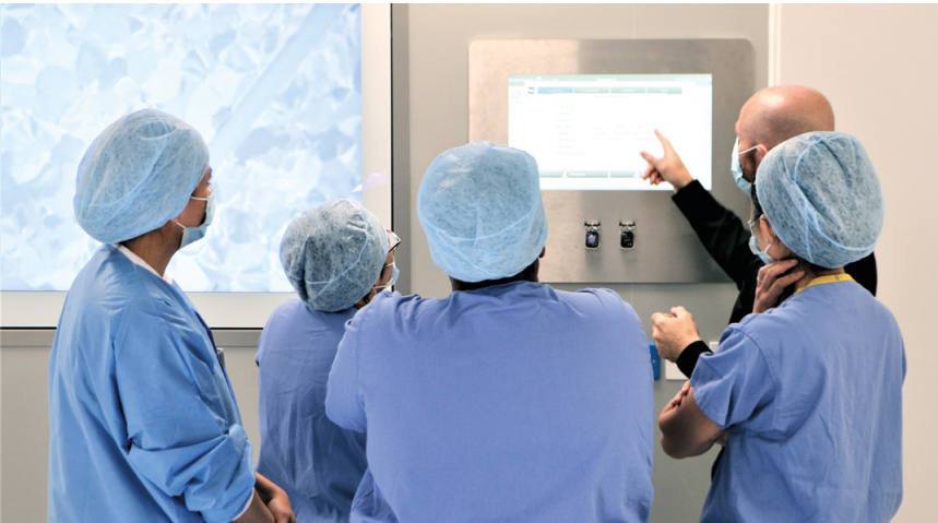
Merivaara's high capacity OpenOR™ integrated theatre solution installed at Epsom Hospital
